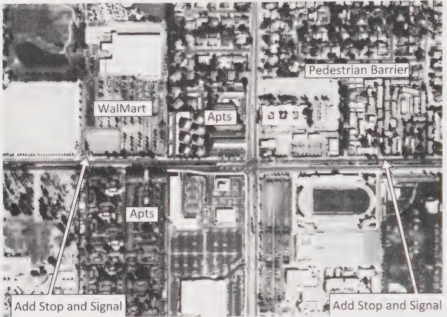
Figure 15-2 Opportunities to improve pedestrian and transit environment. Kings Canyon Road and Peach Avenue, Fresno, California.
